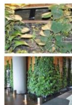
Figure 1: Plants and soil held by wire mesh, watered by small tube with gravity-fed drip system.
