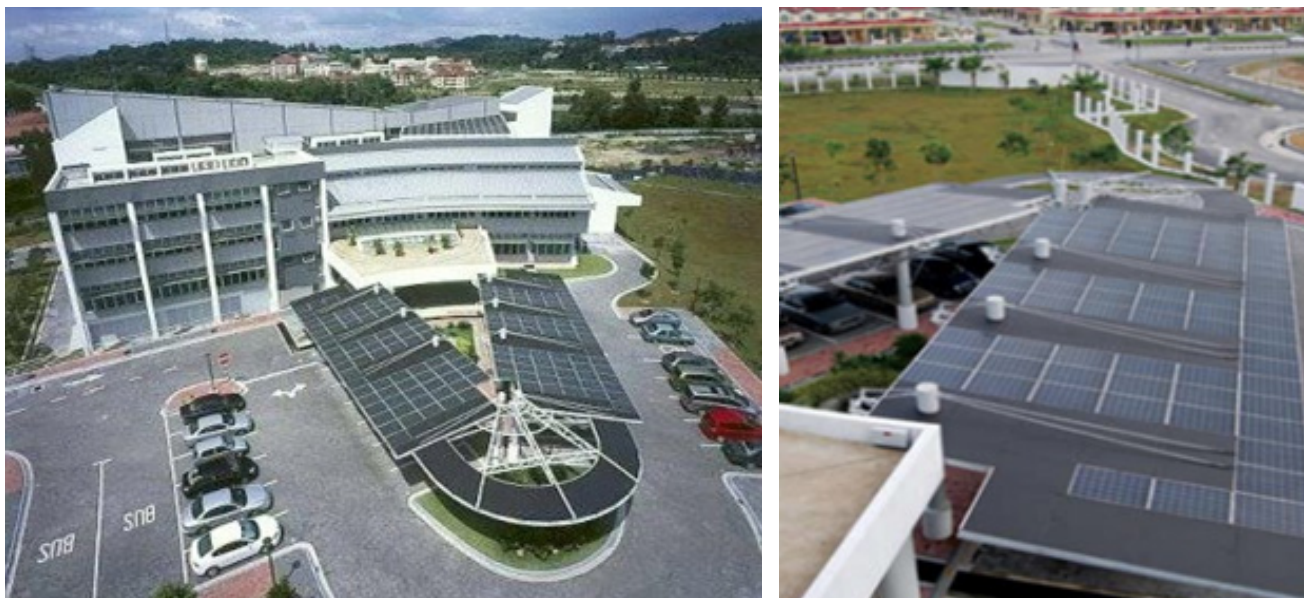
Foto 23: Bangunan tenaga sifar yang berkonsepkan Building Intergrated Photovoltaic (BIPV), Malaysian Green Technology and Climated Change Centre (MGTC)
