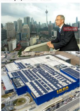
IKEA Cheras – 1,002 kWp
